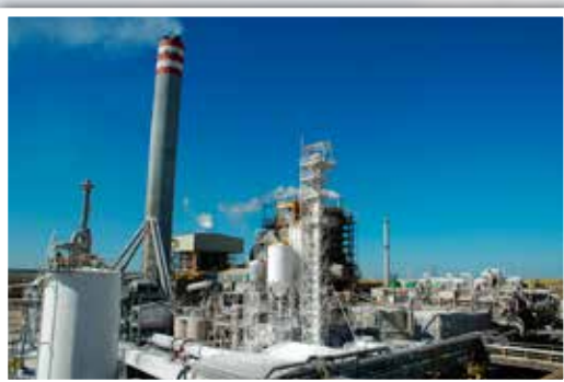
ENCE facilities in Huelva, Spain
